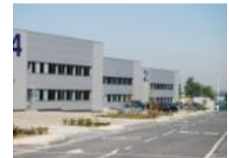
The Interchange, Swanley, Kent
