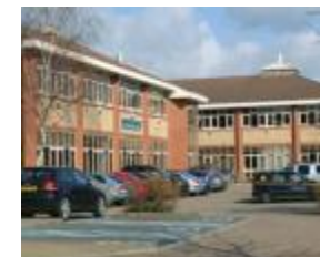
Britannia Road, Waltham Cross, Herts
